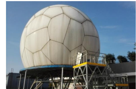
Digital Phased Array Antenna far Field Testing Laboratory
